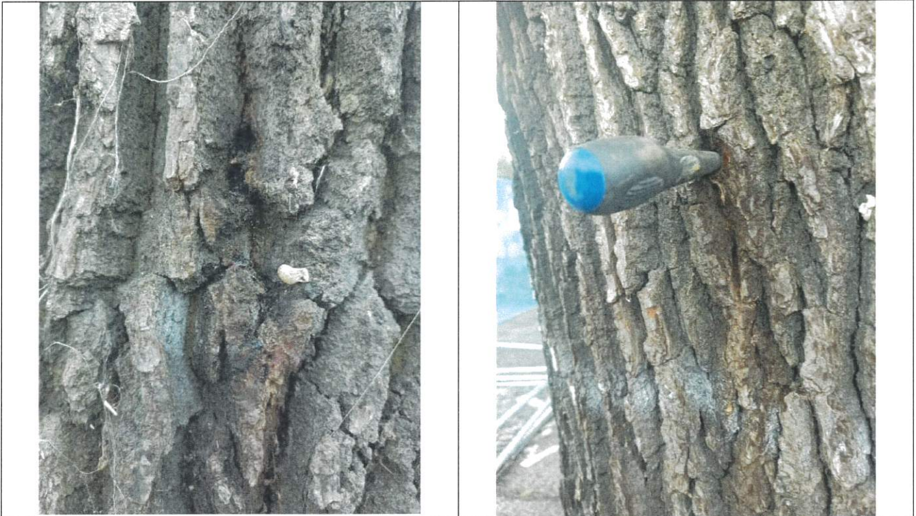
Figure A3.3: 12mm diameter drill hole with encircling exudate and 10cm screwdriver inserted into the hole on the eastern trunk.
